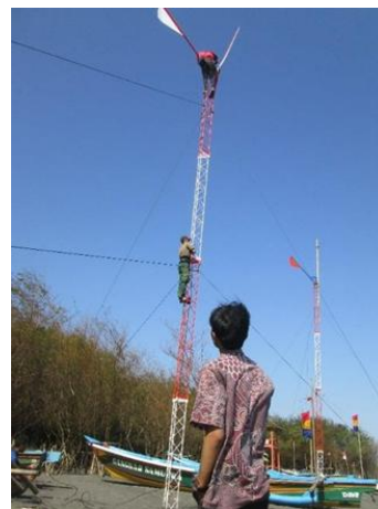
Fig. 2. Wind Turbine Installation
